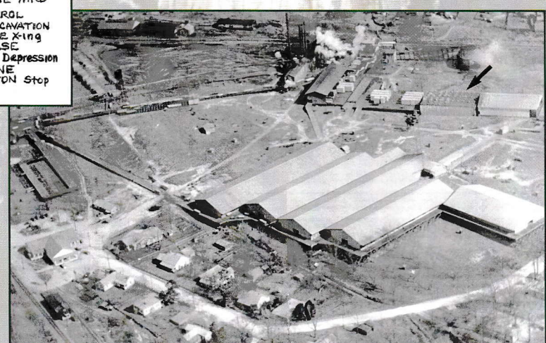
General aerial view of millsite and some surrounding company housing. Extraordinary characteristic is the huge lumber storage shed which was the predominate feature in the trail area and of the entire plant site, being much larger than any other buildings then or now. It is easy to observe that the shed was built on pilings (some as high as 20') in order to create a level floor out across the sloping and irregular topography. The shed was dismantled in 1955 and no traces of it are evident. (old dry kiln in operation = ←)
