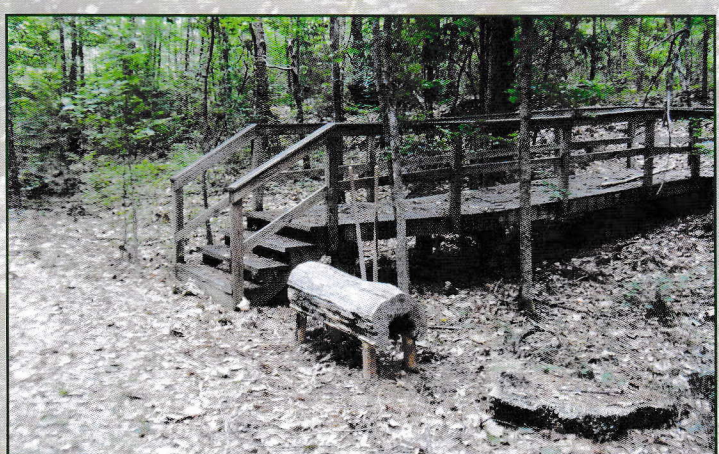
UPPER ROUTE: bridge and bench
