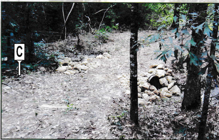
WATER QUALITY: drainage and bridging...sign describes water collection and drainage and how use of a culvert is one method to cross the water course without damage, and how consideration should be given to sizes and other types of installations.
