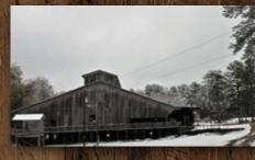
Beside the Planer Mill is its Power Plant. Three huge boilers provided steam to power a Corliss engine that rotated
