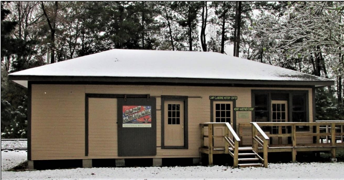
Henry Hardtner's office and carriage from Alexandria now houses two significant exhibits at the Southern Forest Heritage Museum. One includes Hardtner's office, typical of an early 20 th century lumberman, and exhibit material about his contributions to forestry. The other, the Camp Claiborne History Center, has focus on the role of lumbering and forestry in the World War II effort. The building has been restored to help continue an understanding of Hardtner's legacy to the South.
